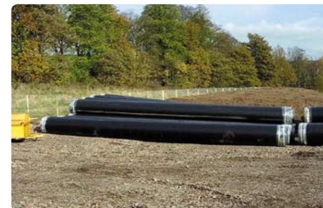
Fig. 2: Pipe lengths made from Hostalen CRP 100 black (PE 100), diameter 1100 mm, manufacturer KWH Pipe
